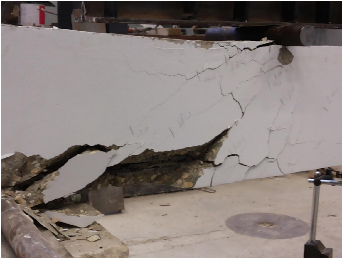
Figure 5: Beam SSB at failure stage.
