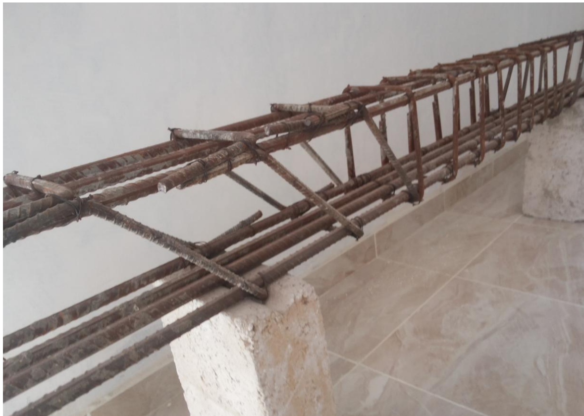
Figure 2: Steel cage reinforcement of the beam reinforced with spliced swimmer bars, SSB.
